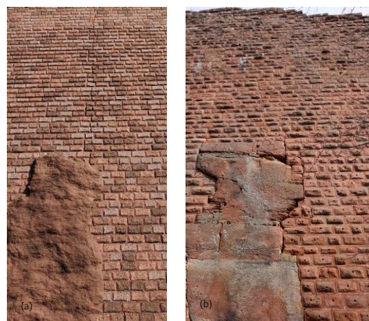
Figure 4. (left) Rendering of the restitution of the Wasenbourg castle (procedural material of a block with a rusticated stone with holes in sandstone); (right) Image of the ruin of the Wasenbourg castle (block wall with rusticated sandstone holes)
